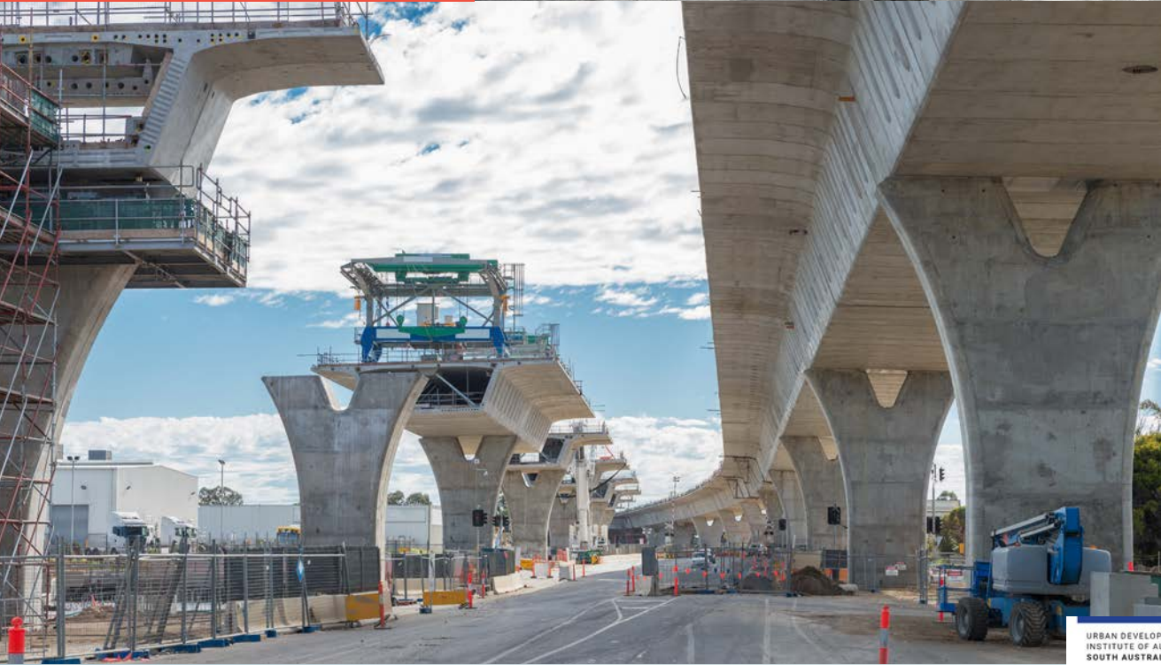
King William Road redevelopment
