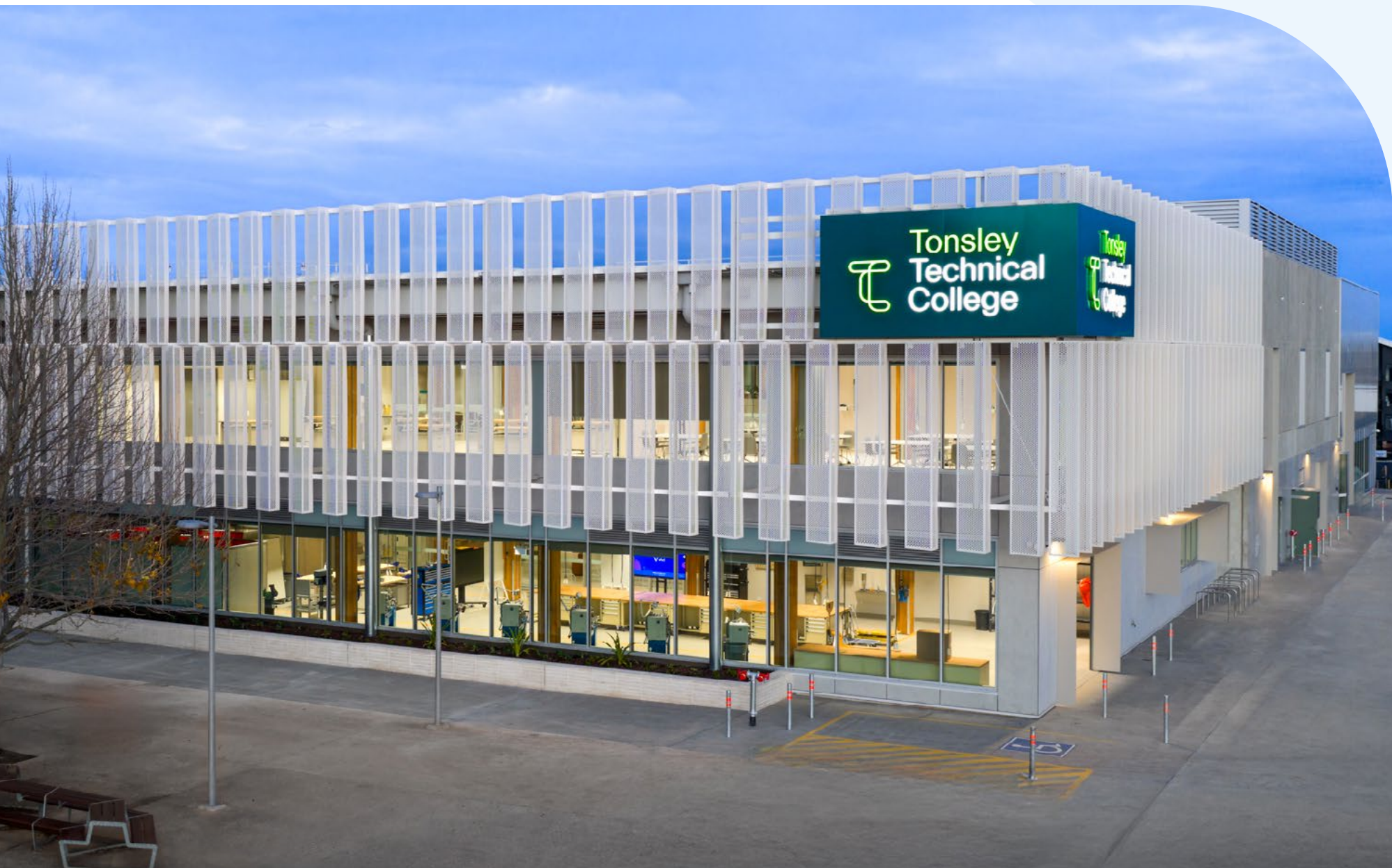
Tonsley Technical College and Factory of the Future Image courtesy of Sarah Constructions
